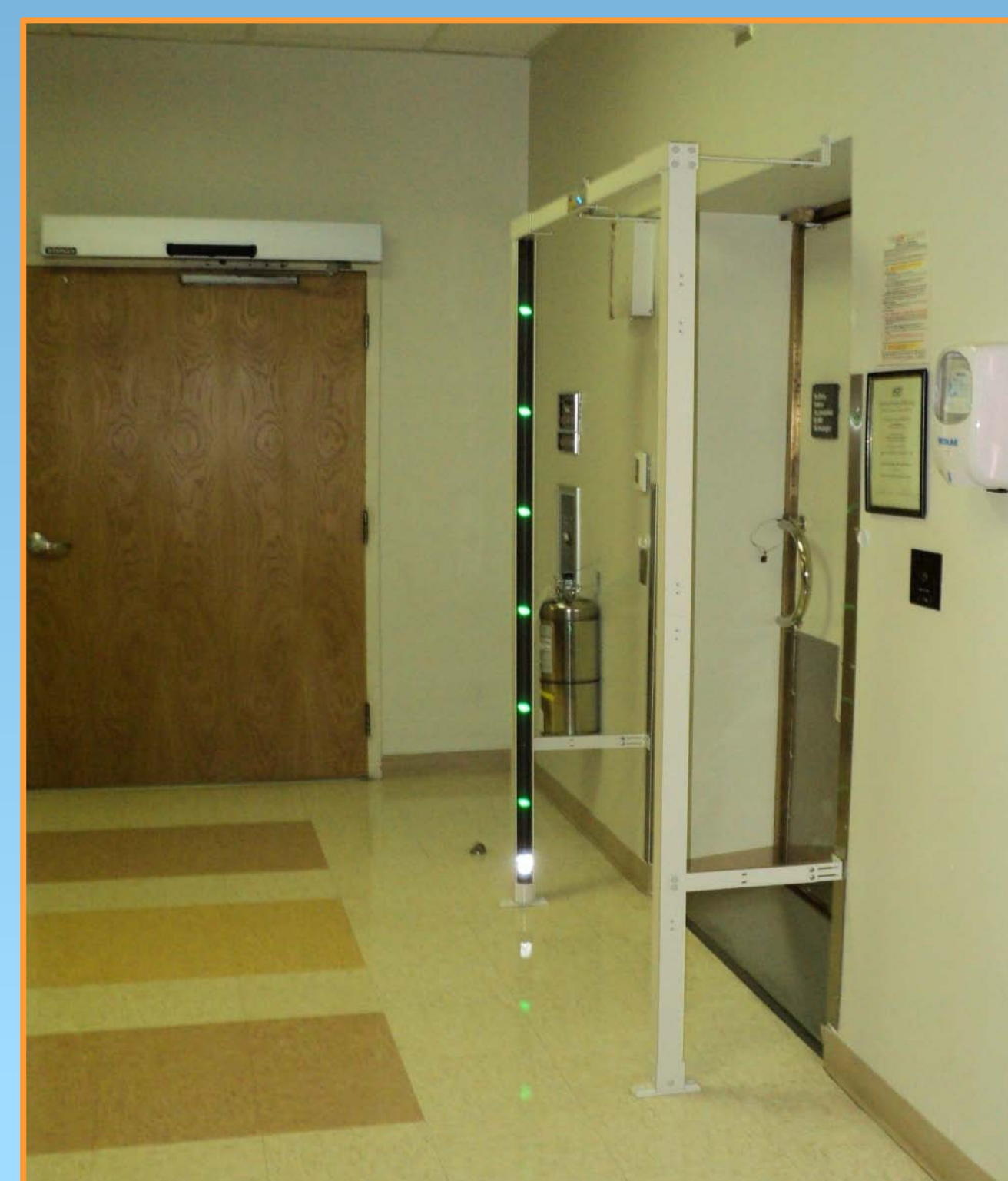
Figure 1. Ferromagnetic detector offset from wall.
