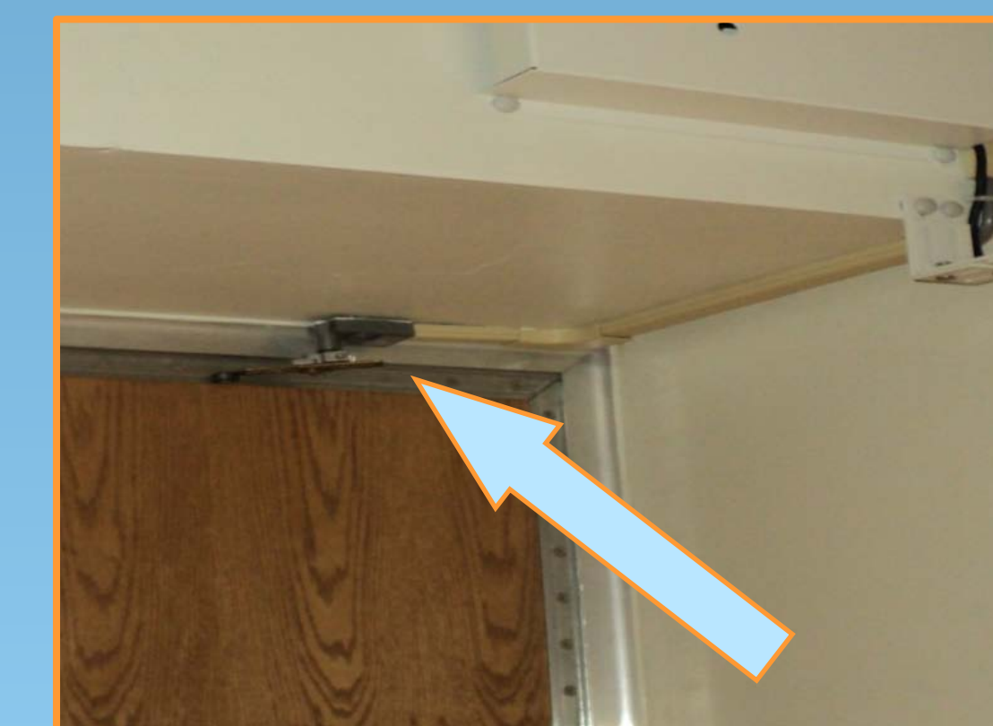
Figure 3. Door switch which only activated the detector when the MRI door was open.
